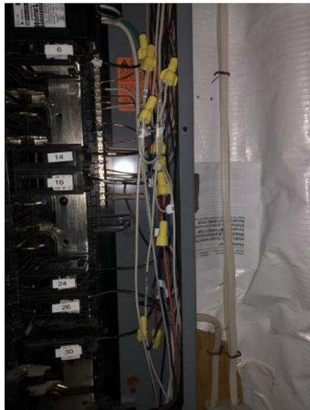
At the transfer switch end I originally ran the Romex from the floor joist into the transfer switch. While functional it didn't meet code. I had 28 inches of unsupported wire.
